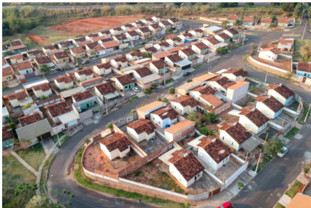
Aerial view of construction site of standardized houses of the Minha Casa Minha Vida Program, in Pompeia city, of the São Paulo State, Brazil. Source: Adobe Stock Images, AlfRibeiro
